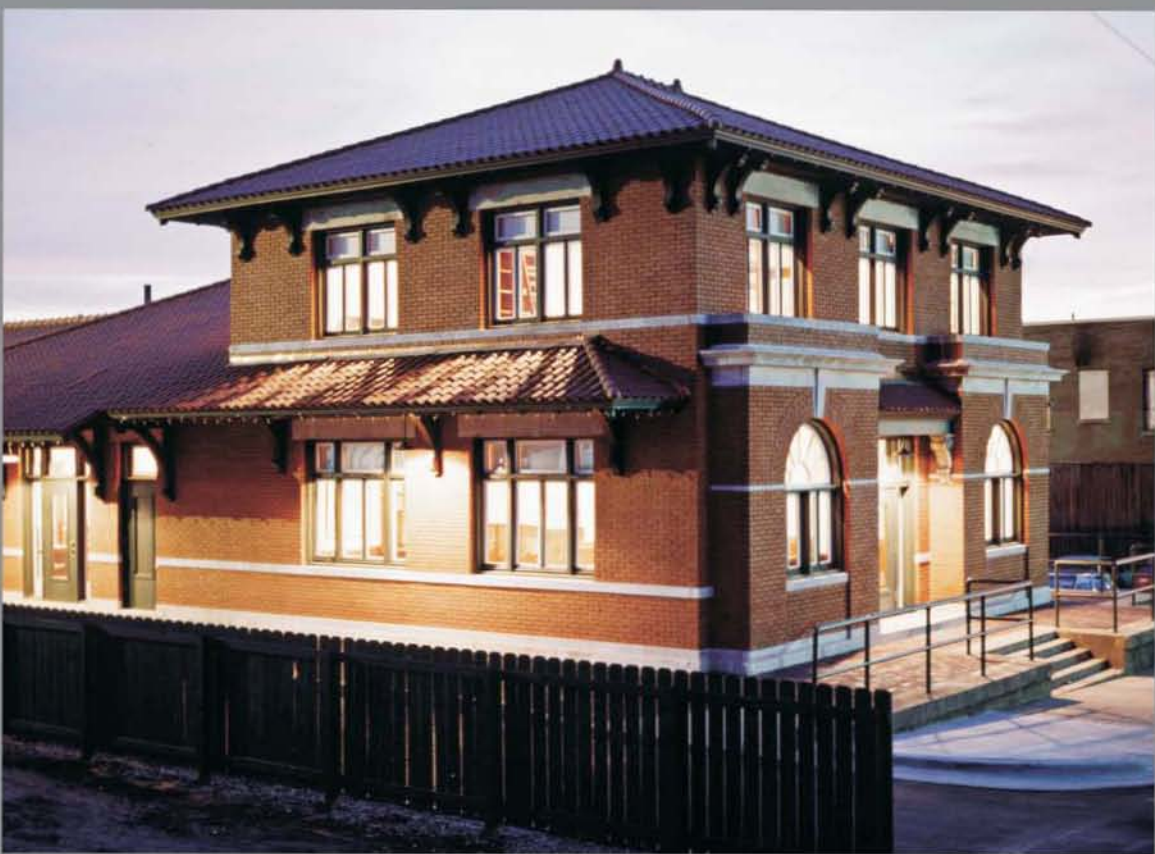
The Missouri-Pacific Train Depot, a part of the Delta Cultural Center Museum, is located in Helena, Arkansas. The Train Depot was named to the National Register of Historic Places in 1987.
